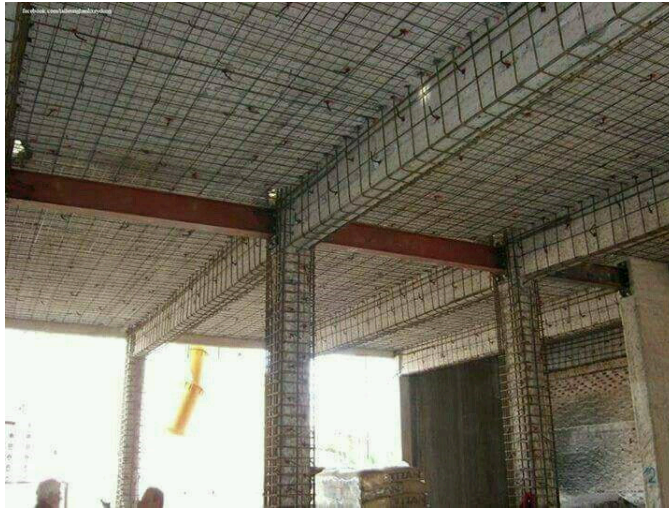
Fig: Diaphragm strengthening by steel sections
