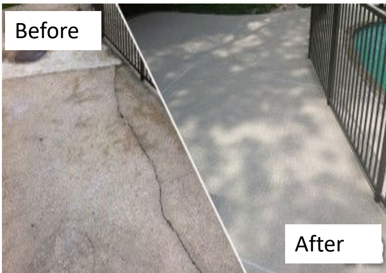
Slab repaired by concrete overlay
