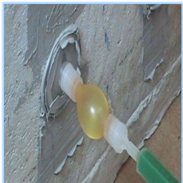
Fig: repair of damaged columns with sight crack (1. Cracks 2. Injection ports)
